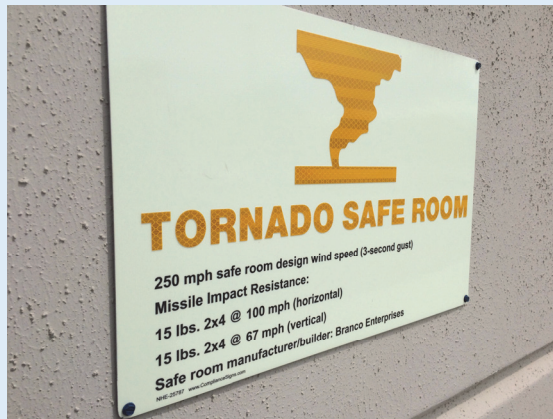
Figure 3-1 Tornado safe room placard.
